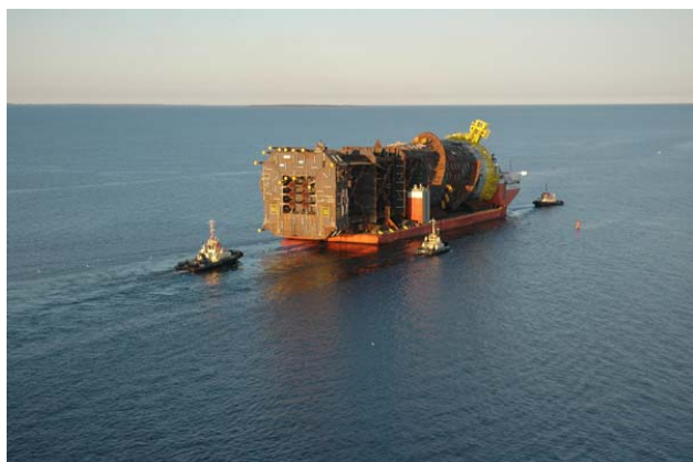
Figure 5: Spar of Perdido platform, getting moved to position in the Gulf of Mexico (from Canty, 2008).
