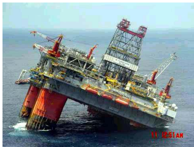
Figure 4: Thuderhorse platform, after hurricane Denis hit it, (Leduc, 2006).
